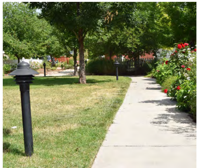
These full cut off bollards only direct light down at the path.
